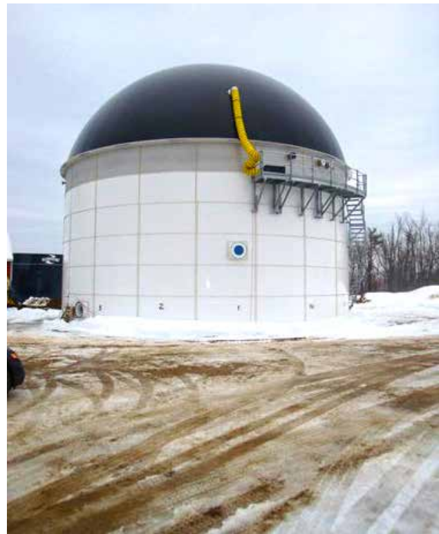
Anaerobic digester at Jordan Dairy Farm in Rutland, Mass.
