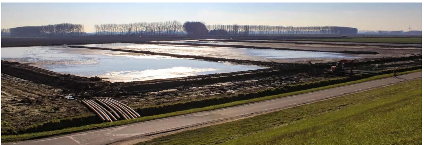
Digestate (Sludge) Drying Bed. Photo Courtesy of Judd and Judd Ltd.
